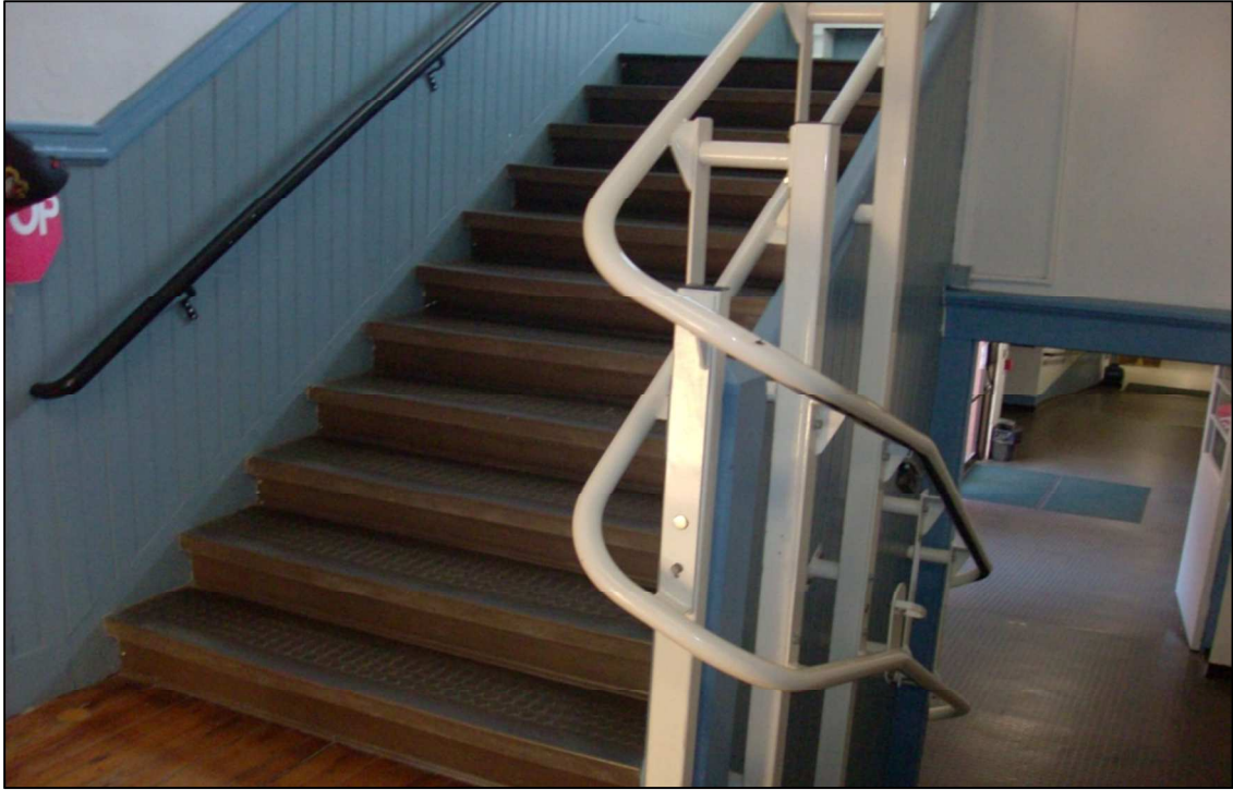
Track for stair lift in original section of school.
