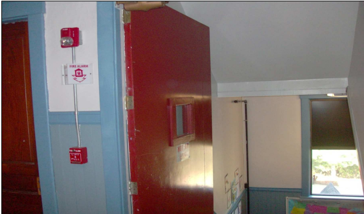
Large heavy fire door at top of stairwell in original section of building.
