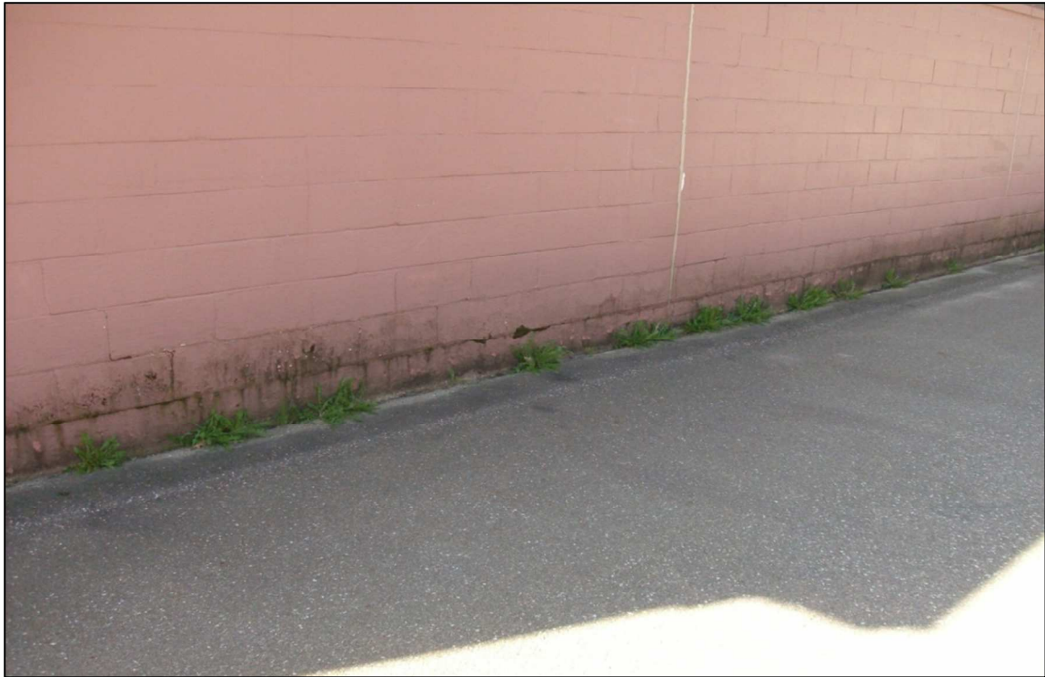
Mold/mildew growth on north side of gymnasium from roof runoff splash back.
