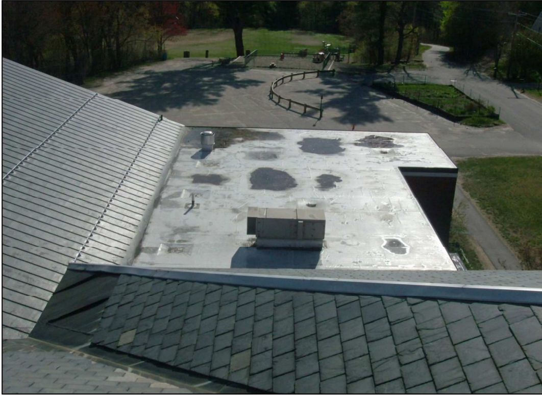
Looking east from original building toward the 1970's addition. Note metal edging along slate roof, water ponding on 1970's TPO roof, and metal roofing with snow guards on gym to the left.
