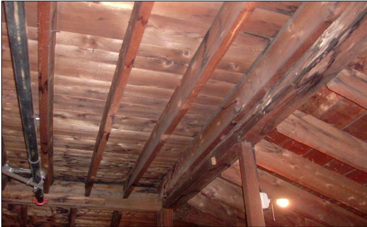
Typical wood framing in the attic. Wood staining may indicate past leakage.
